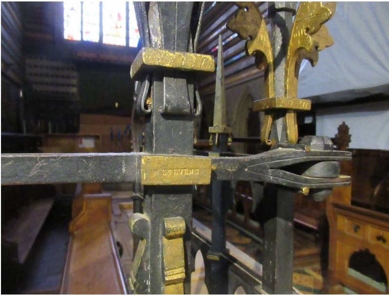
One of the Cliveden guys pointed out to Ken the name of Stevens on the ironwork on the dwarf wall. It appears again on the other side. I have no idea who Stevens was as the iron work is attributed to Leaver.
