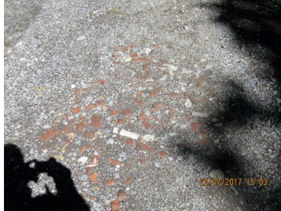
Figure 13 Brick hardcore in lane
