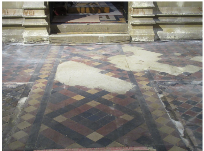
Considerable damage to the floor under the platform. In the photo on the left you can see a tile smashed into little pieces. It seems as though something very heavy was dropped on it as the floor is even indented at that point.
